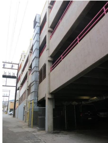
**Figure 8.** HVAC air intake at the rear of the parking garage.
