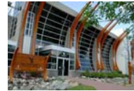
The Two Rivers Gallery is the major art gallery in the Central Interior of British Columbia, and serves a larger region. The facility was built for a cost of $5.2 million, with $1.25 million raised through art gallery Capital Campaign.
