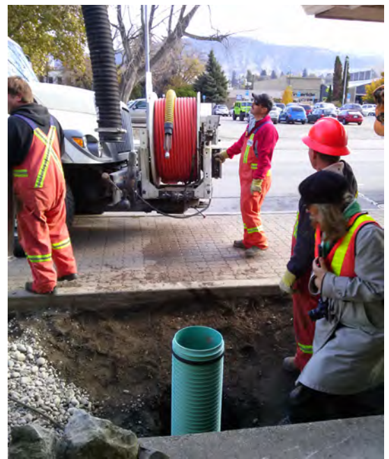
Image 3: Installing the well casing
