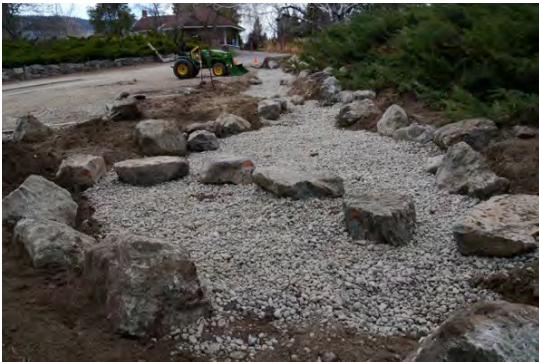
Image 4: Dry creek bed was filled with gravel and large rocks were selectively positioned
