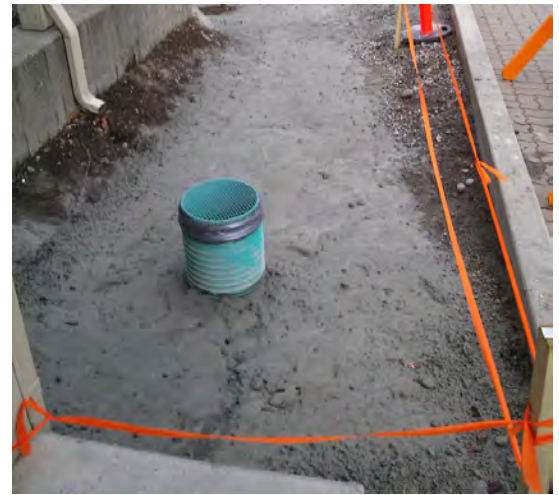
Image 4: Amending soil with clay barrier
