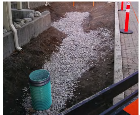
Image 5: Irrigation ditch and drain rock
