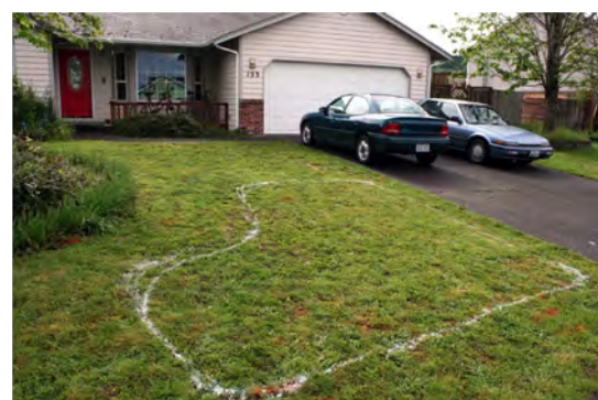
Image 6: Using spray paint to lay out garden area
