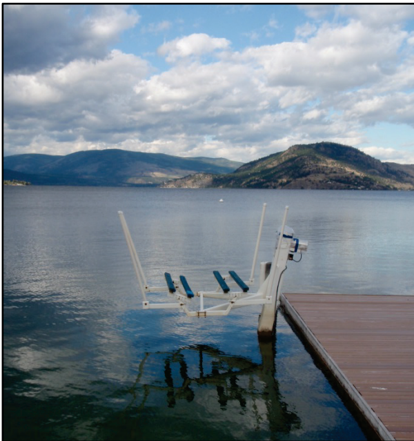
Photo 2: Lake intake location (white buoy).
