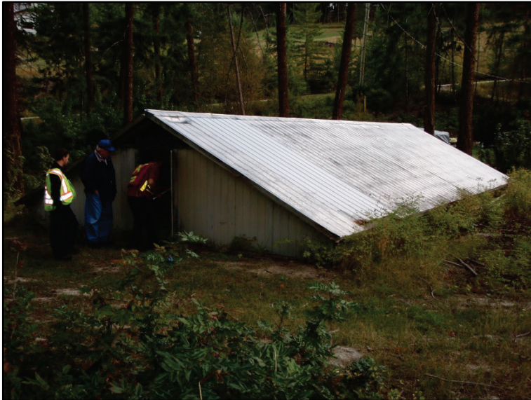
Photo 11: Reservoir roof structure.
