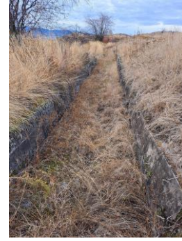
Figure 10: North view of concrete walls in the canal/flume
