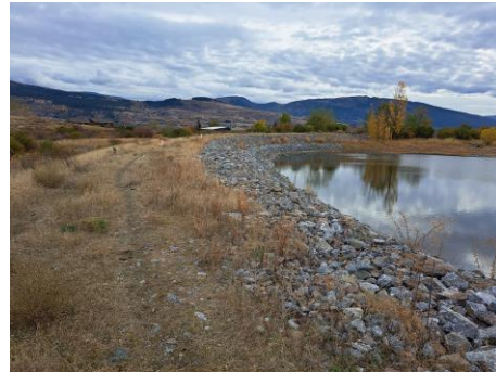
Figure 16: View east along top of dam, cattle fencing visible along the toe of the slope on north side
