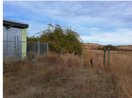
Figure 18: View north of existing trail entrance with small cattle cate adjacent to chlorine plant
