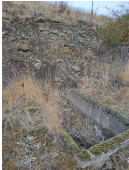
Figure 11: View of canal infrastructure apparently draining out of Wetland 5
