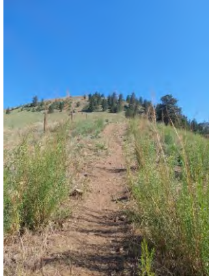
Figure 16: View of existing trail with 30% grade and a loose trail surface to be rerouted.
