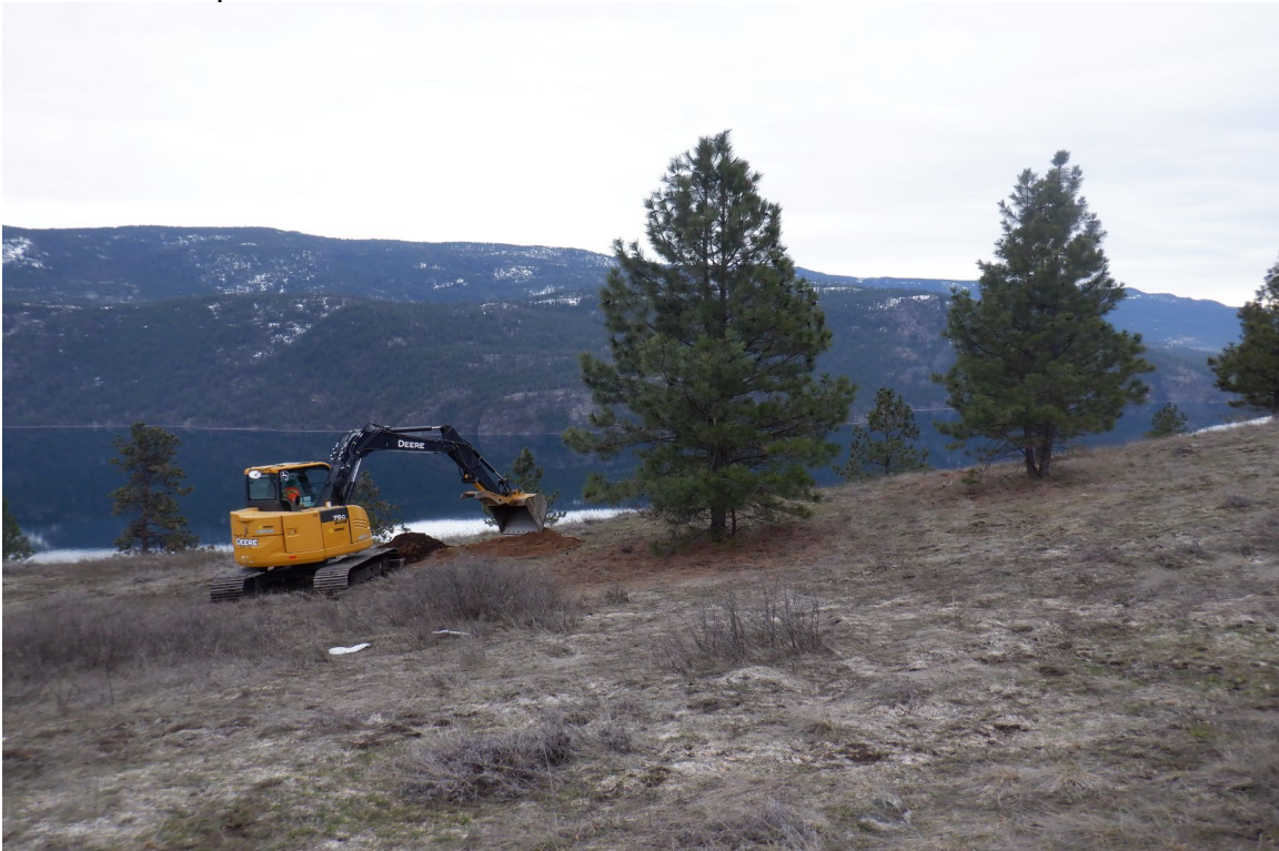
Photo #2 – bottom station testpit 2.0m deep with sand & gravel
