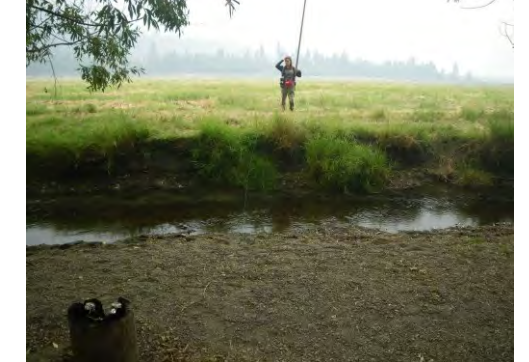
Looking across the channel at the left (south) bank.
