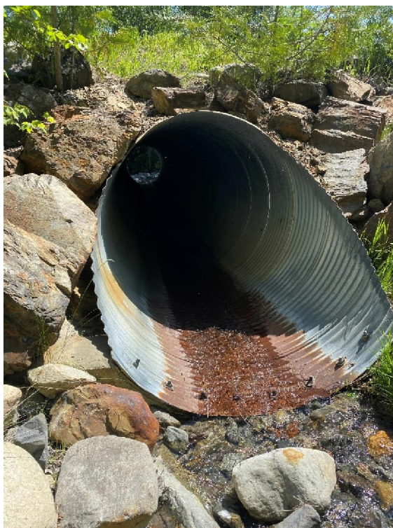
Photo 8 Upstream Inlet of the 1600 mm Culvert at Ladyslipper Road
