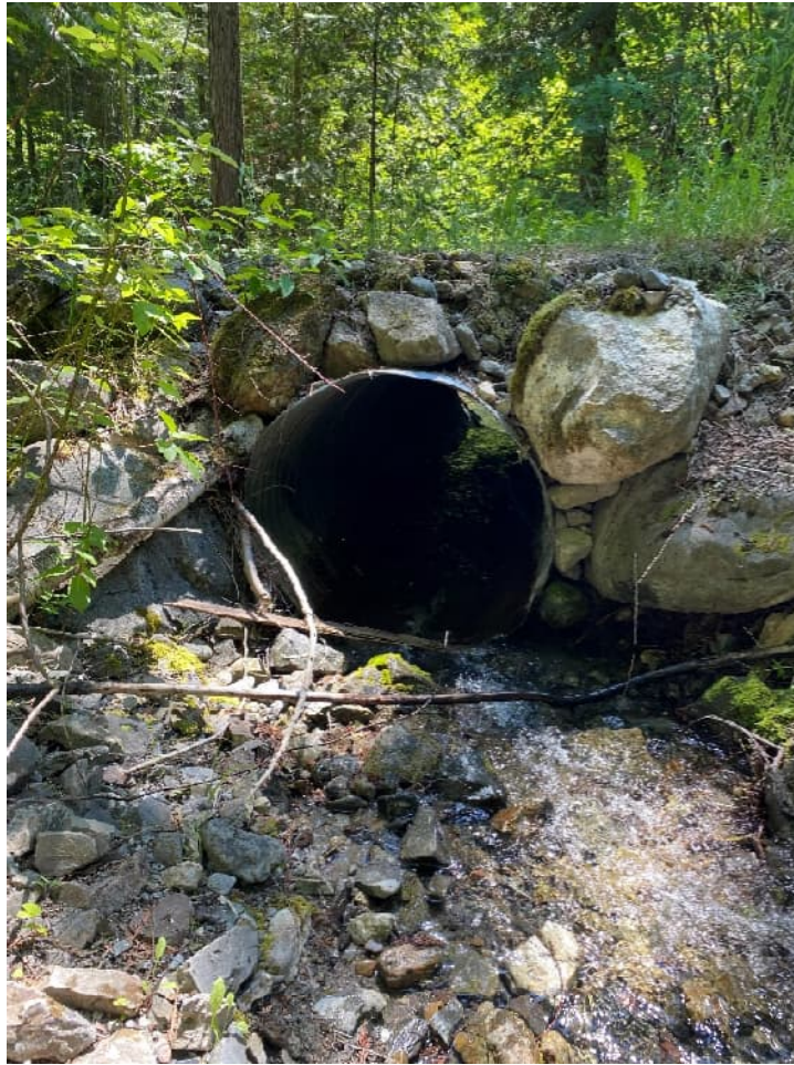
Photo 9 Upstream Inlet of the 900 mm Culvert
