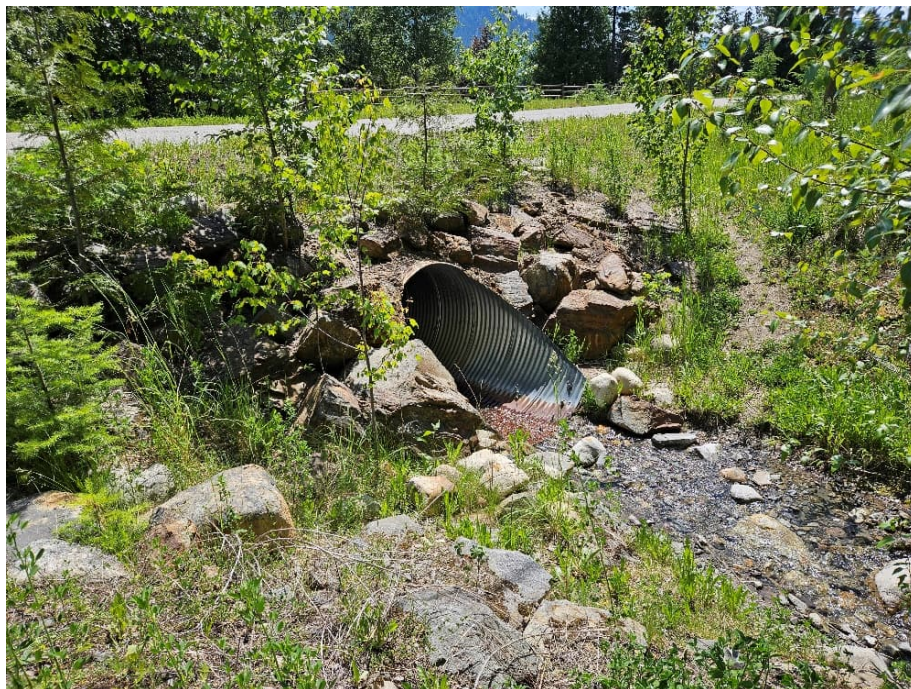
Photo 7 1600 mm Culvert at Ladyslipper Road
